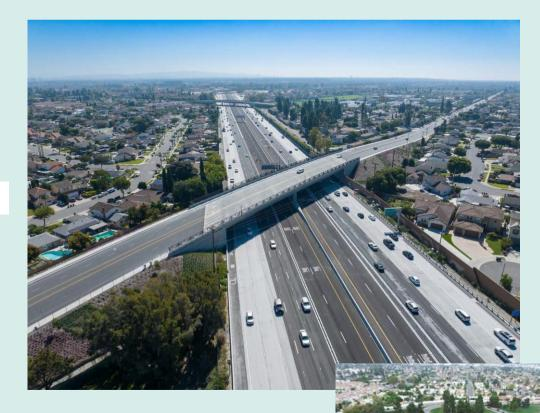
Following sustainability criteria, 710,000 tons of concrete have been recycled, reused for the base layer of the new lanes. In addition to reducing emissions, the project will improve journey times by removing bottlenecks. Travelling time is expected to be cut down by half for nearly 400,000 daily drivers.
